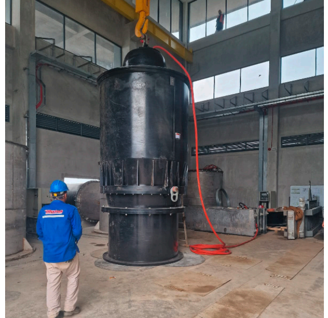
Bedford's 10,000 l/s SAF pump during installation on site
